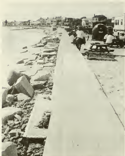
Bicentennial Park: Seawall gap filled in by DPW
