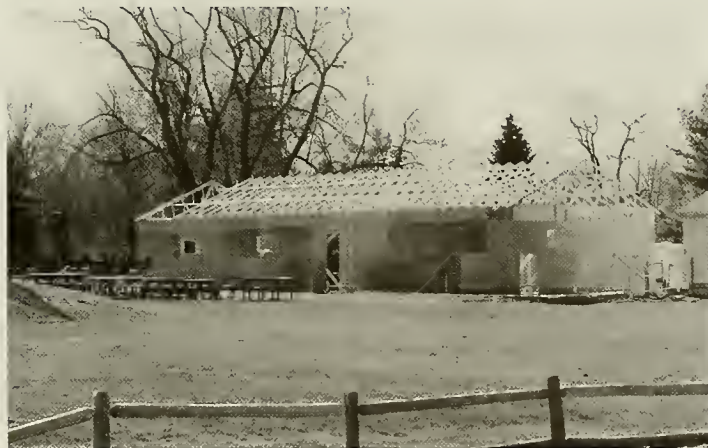
The new Tuck Building under construction.
