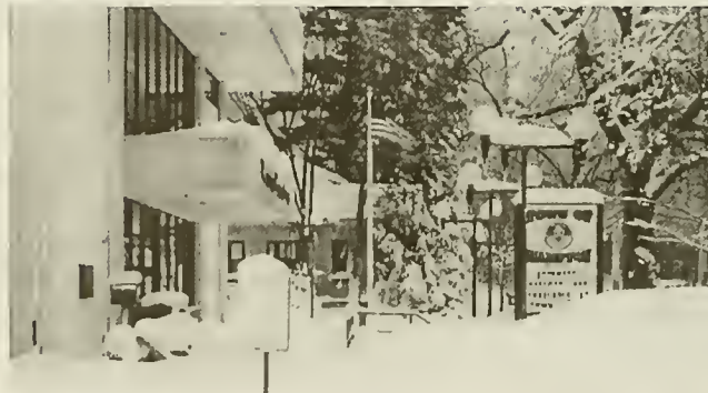
The Town Office in the aftermath of the March snow storm.
