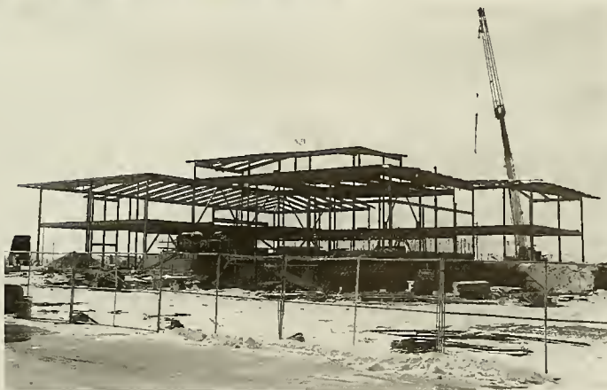
The framework of the new police facility – January, 2004
