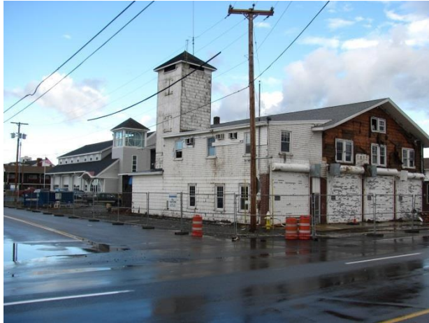
(Ashworth Ave Station on demolition day)
