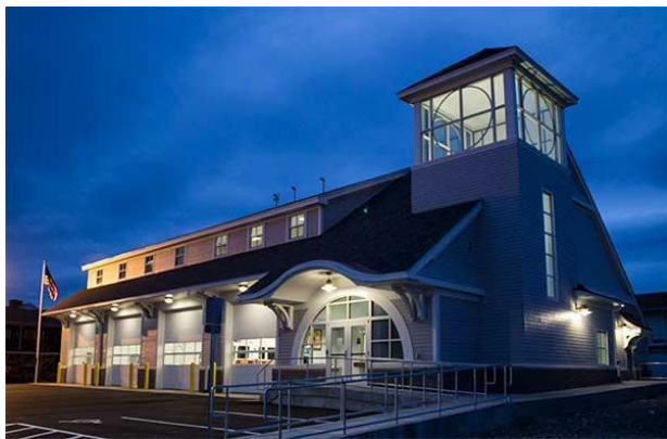
(Completed Beach Fire Station)
