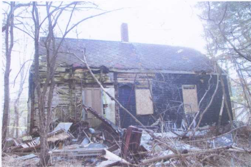
A view of the house from the rear. The backside of a plaster wall in the kitchen became visible when the addition which contained the sink and washing machine collapsed. The asbestos shingles have been removed.
