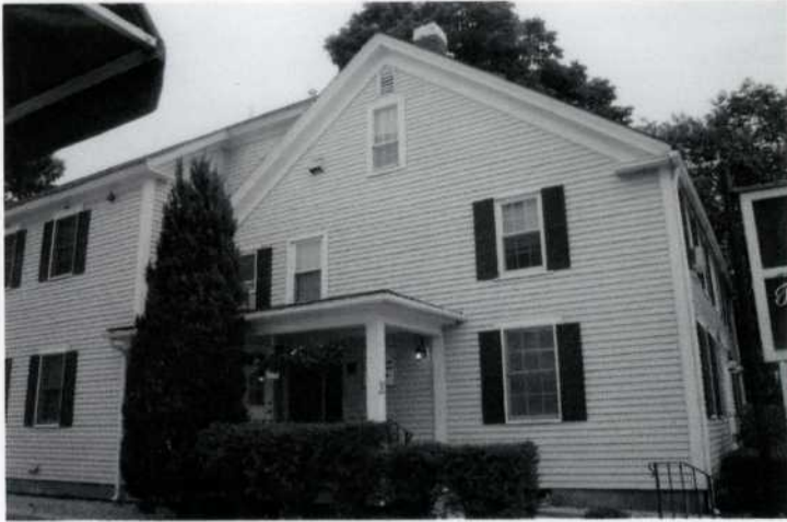
A view of the building from the west.
