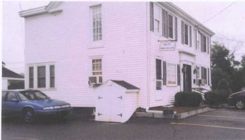
• A view of the building from the west. The front of the building faced south despite the location of any roads, a common feature of early construction in Hampton.
