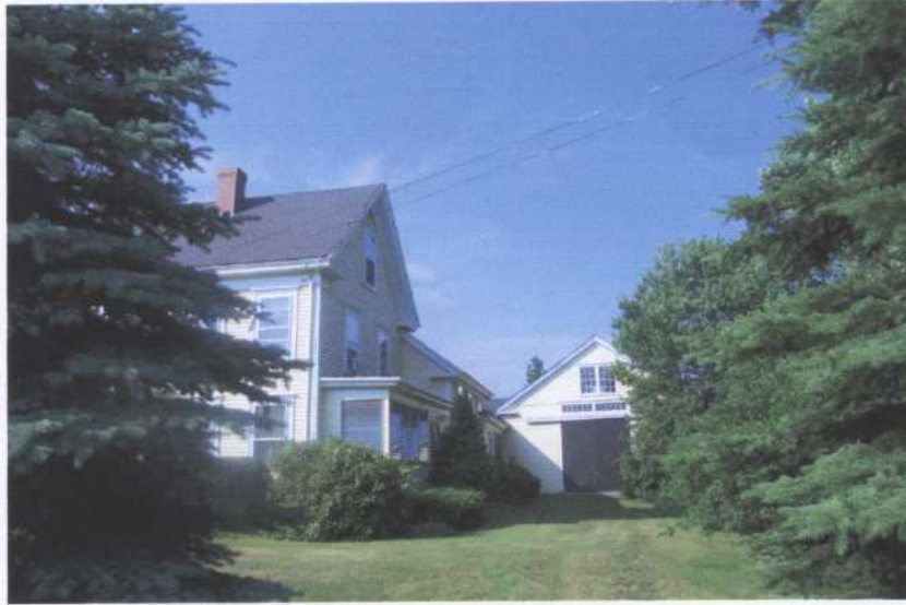
A view from the south showing the barn.
