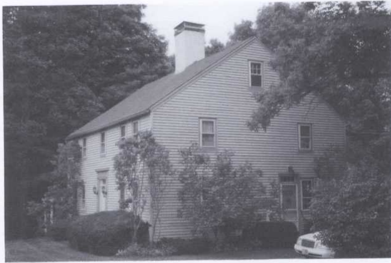
View of right side of house.
