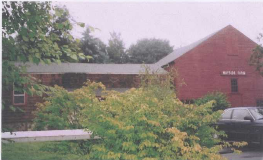
View of additions from the house to the barn.
