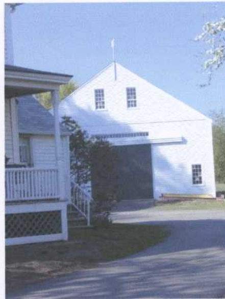
View of barn along east side of house.
