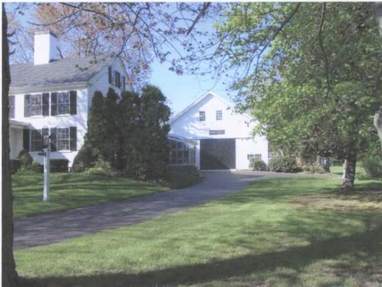
View of barn behind house.
